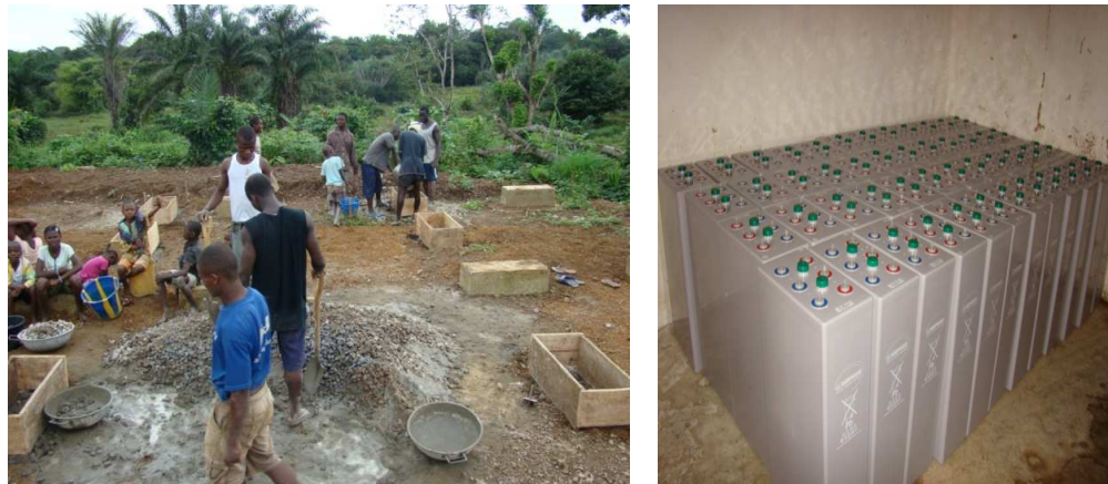
Figure 17a - Pujehun Growth Centre 11 kW PV system in construction
